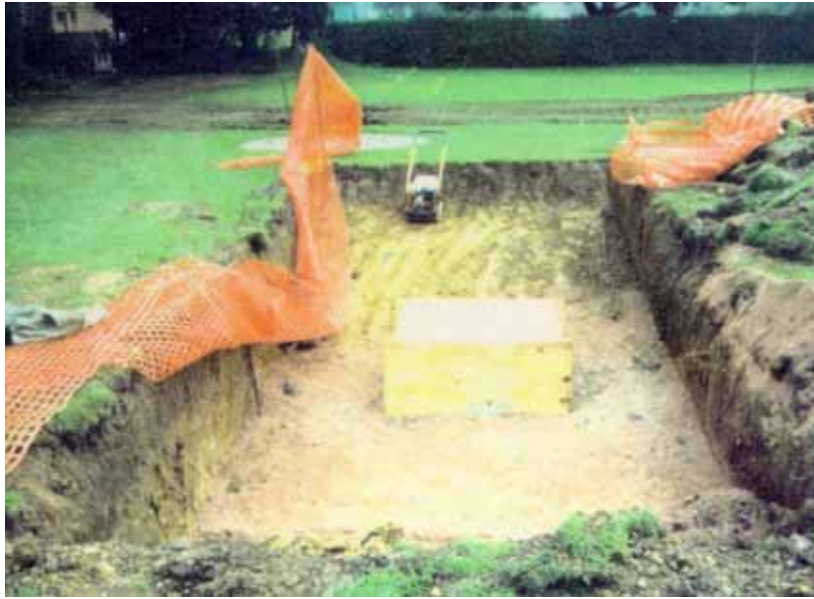
Area 7: Sandpit with cast concrete blocks.
